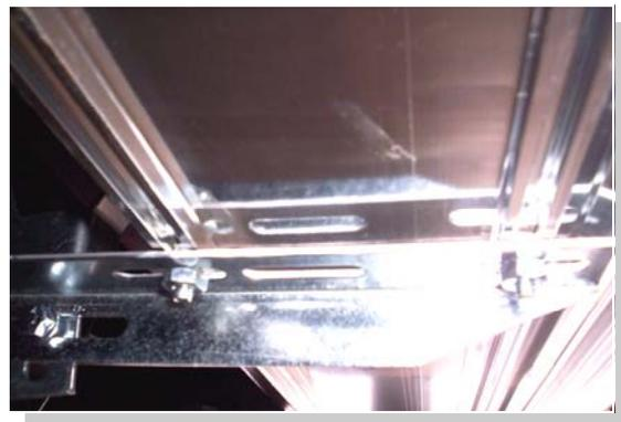
Attach 3124F to FL217 using 5/16" nut and bolts, Snug but don't tighten. Place the board on the brackets with the bolts through the slots. Fasten with 1/4" nuts.
