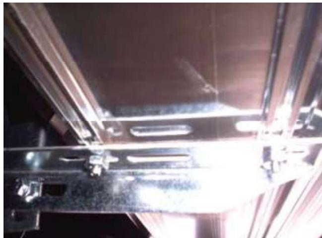
**Step 11:** Tighten all remaining nuts and bolts. Make sure every one is tight to reduce rattling.
