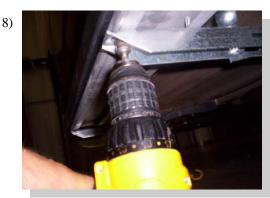
With board level and properly aligned, attach to the brackets with 3/4" long self drilling screws.
