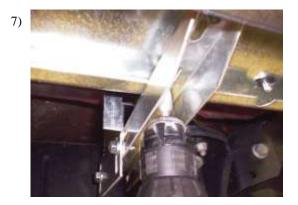
Place the board on the brackets. Attach with self drilling screws. You may need to adjust channels for level and Straightness.
