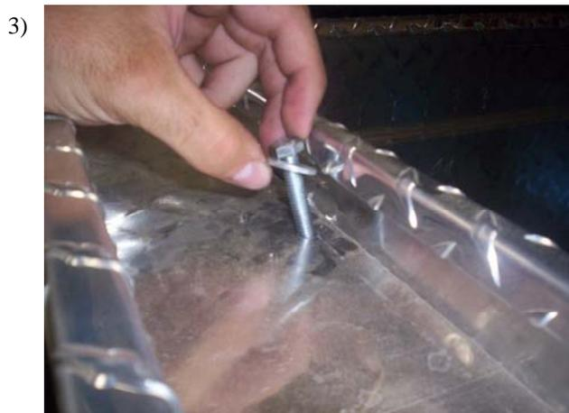
Insert 5/16" bolt and washer from inside of tool box through drilled hole.
