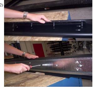
Using a 5/16 drill bit, drill a hole into the board through the holes in the step (<u>Use the dimples on the top</u> of the board for drilling locations when dimples are present. They may not align with holes in the steel plate.)
