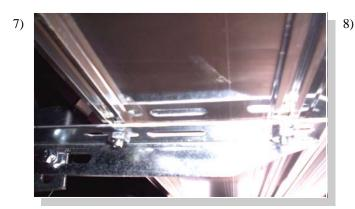
Place the board on the brackets with the bolts through the slots. Fasten with 1/4" nuts.
