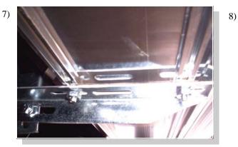
Attach 3124F to FL217 using 5/16" nut and bolts, Snug but don't tighten. Place the board on the brackets with the bolts through the slots. Fasten with 1/4" nuts.
