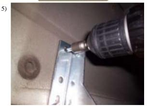
At remaining locations install two self tapping bolts through slot in FL223 and FL232 (**Different BRKT shown**)
