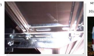
Attach 3124F to FL223/FL232 using 5/16" nut and bolts, Snug but don't tighten. Place the board on the brackets with the bolts through the slots. Fasten with 1/4" nuts.
