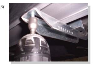
Place the board on the brackets. Attach with #14 self drilling screws.
