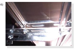
Attach board to brkts by inserting the square head bolts through the slots in the brkt. Attach1/4" flanged nuts to square head bolts, but don't tighten at this time. Center board left to right and tighten the 1/4" flanged nuts.
