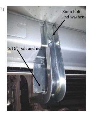
Attach CB71 channel bracket using a 8mm bolt and flat washer into the inpull nut and a 5/16" bolt and nut . **Tighten all bolts.**
