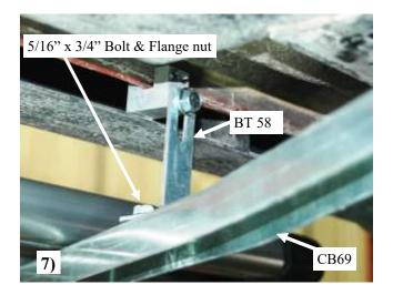
7) Mount the CB69 channel onto BT58 with a 5/16" x 3/4" bolt and flange nuts. **Picture 5**
