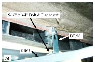
5) Mount the CB69 channel onto BT58 with a 5/16" x 3/4" bolt and flange nuts. Picture 5
