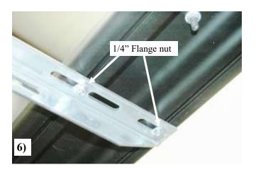
6) Slide (1) hex head bolt into both the front track and rear track for each bracket location.
