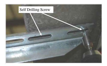
Using self drilling screws attach the board to the angle brackets making sure you are drilling into steel mounting pads. Level board and tighten any remaining loose bolts at this time.
